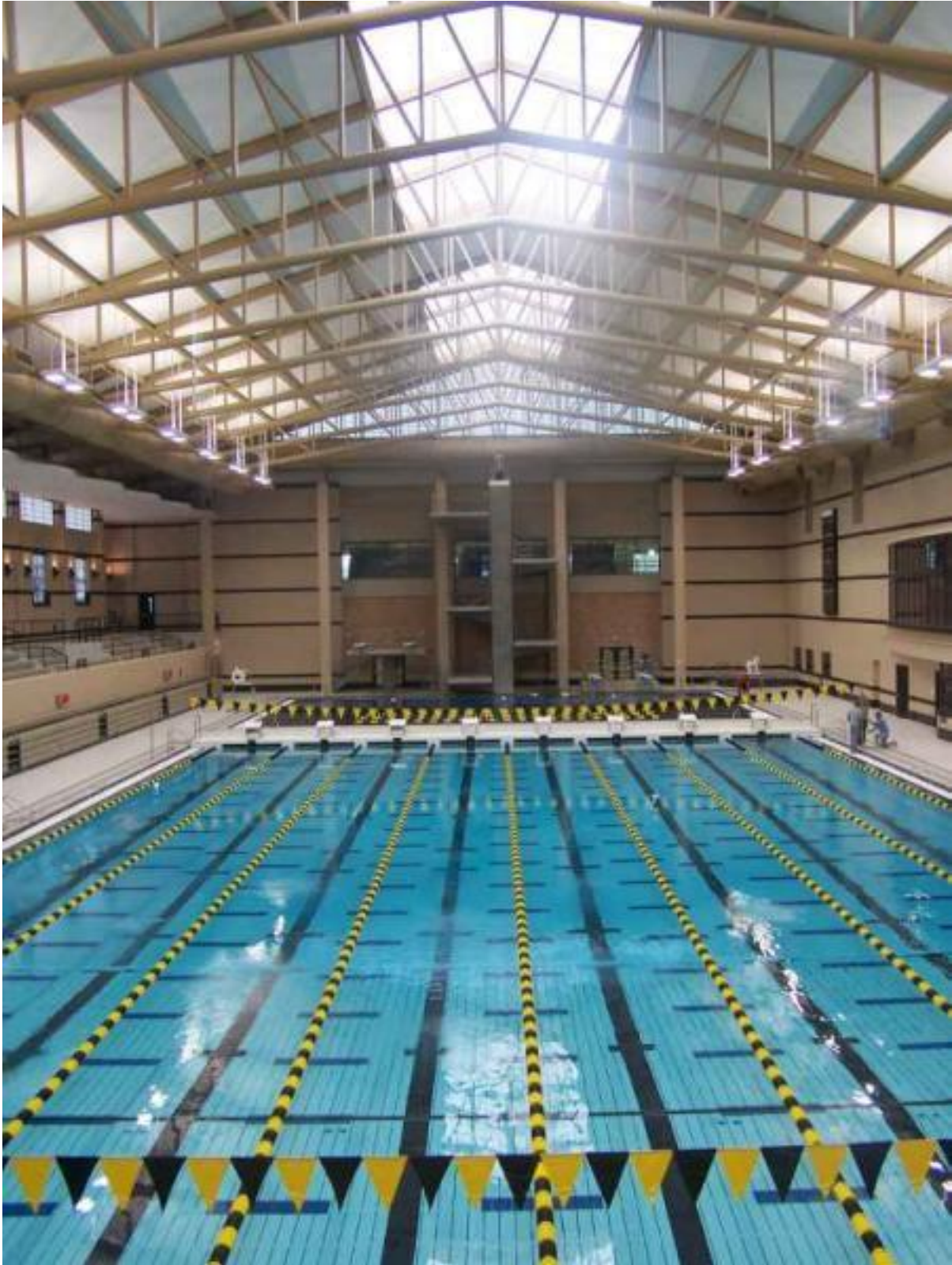
University of Missouri Aquatic Center: Example of Natural Day Lighting
